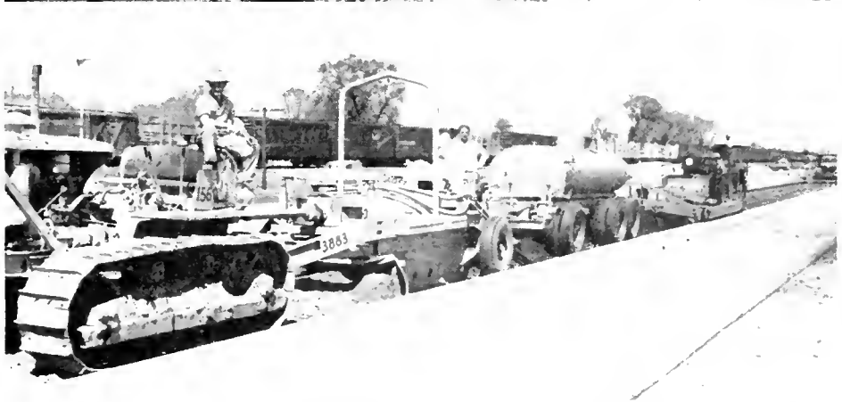
Modern cement treated operation. UPPER—Cement is hauled to project in large truck-trailer combinations from which it is bulked off into smaller distributor trucks. CENTER—Cement is uniformly distributed to the windrow. LOWER—Mixing train follows. Tractor-powered mixer works windrows, adding water from following tank truck. Towed blade breaks down and distributes it. A roller immediately compacts the treated material.
